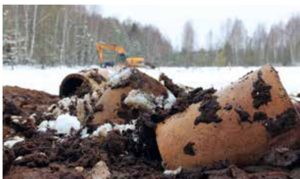
Figure 148. Old asbestos pipes were broken in order to restore water level in the Pūsčia peatland. Photo: J. Sendžikaitė.
