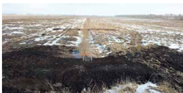
Figure 127. Blocked collective ditch in the Amalva peatland, February 2021. Photo: Z. Sinkevičius.
