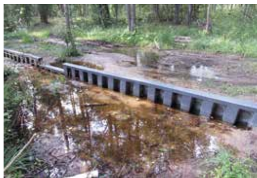
Figure 44. Plastic dam in the Engure restoration area in August 2021, more than half a year after building. Photo: A. Priede.
