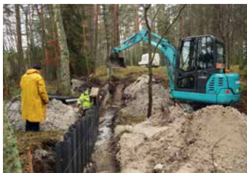
Figure 43. Installing the plastic piling in the Engure restoration area. Photo: M. Pakalne.
