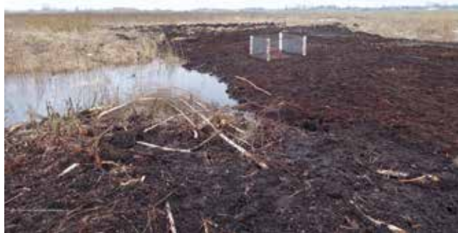
Figure 128. Dam with water outflow construction in Amalva peatland, March 2021. Photo: J. Sendžikaitė.
