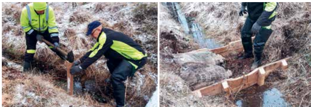
Figure 100. Manually built dams in Wielkie Bagno (winter 2021). Photos: W. Spychala.
