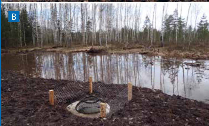
Figure 163. Installation of water outflow embankment (A) with a water outflow construction (B) in Sachara peatland, March 2020. Photo: L. Jarašius.
