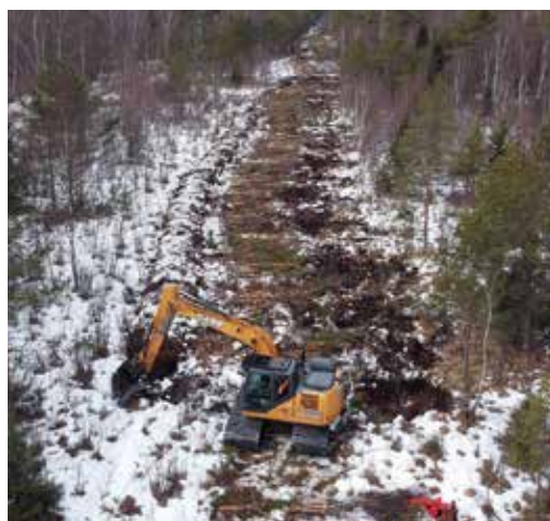
Figure 23. Construction of a peat dike running along the Piirsalu stream. Photo: R. Pajula.
