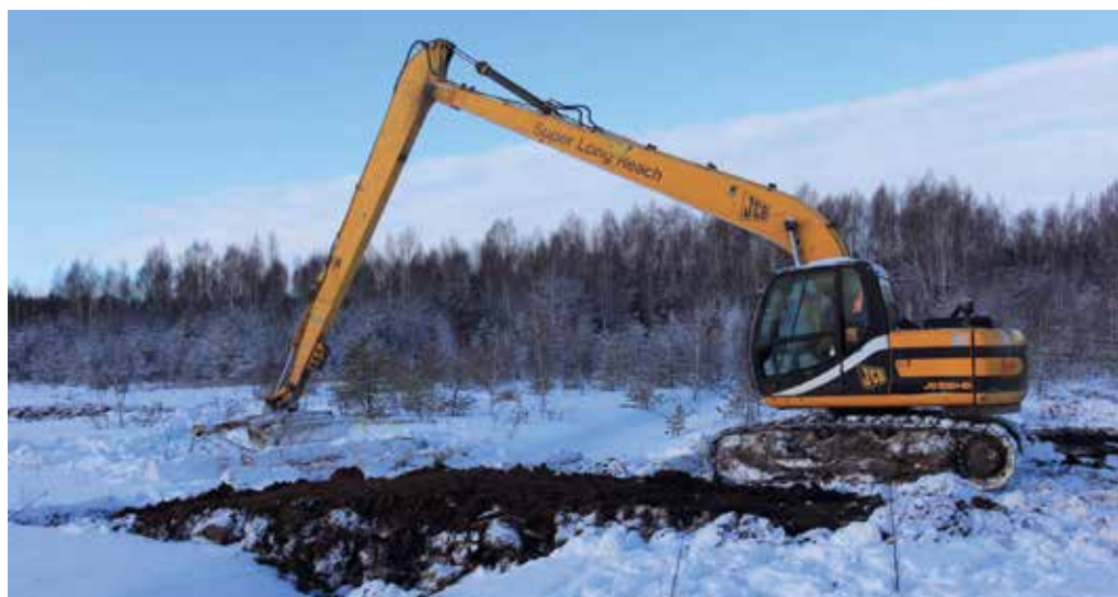
Figure 145. Installation of a peat dam in the Pūsčia area. Photo: Ž. Sinkevičius.
