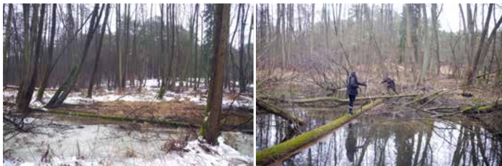
Figure 72. To increase the water level in the Pfauenfließ River, structures like logs, branches and soil material were placed in an irregular manner reducing the cross-section of the watercourse (February 2021). Photo: J. Etzold.
