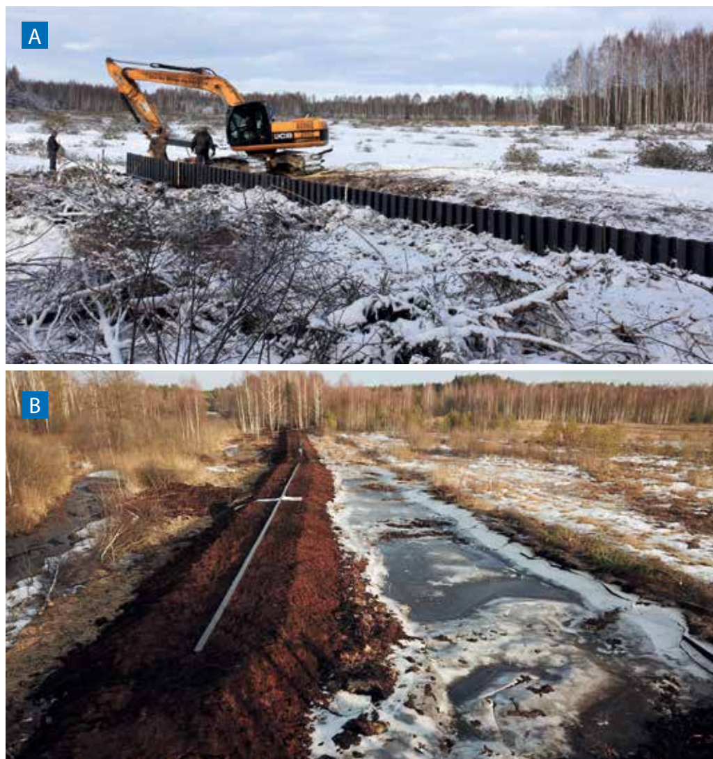
Figure 151. Protective peat embankments reinforced with plastic pile sheets. Construction process (A) and the installed embankment (B), February 2019. Photos: Ž. Sinkevičius.
