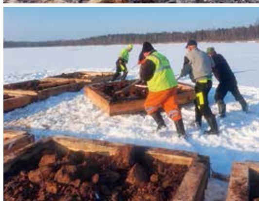
Figure 108. Installation of floating islands, March 2021. Photos: W. Spychala.
