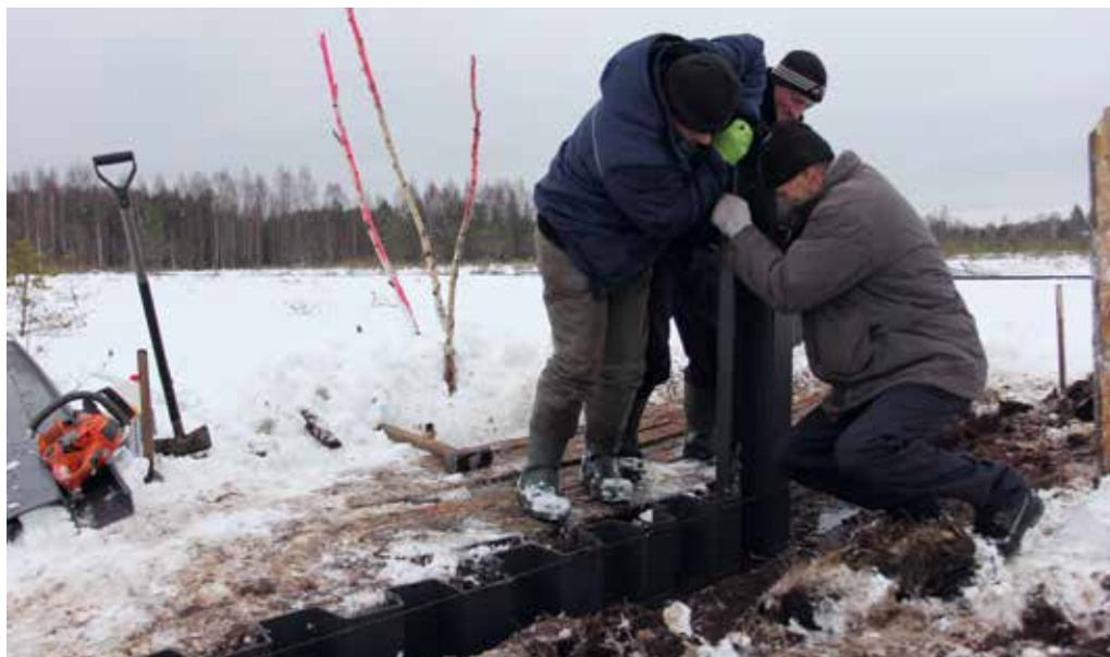
Figure 145. Installation of a peat dam in the Pūsčia area. Photo: Ž. Sinkevičius.
