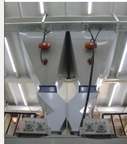
FIGURE 14 New lighting system (occupies less space, does not allow for dust collection, is no attractive for insects, is well protected, and has better light distribution)
